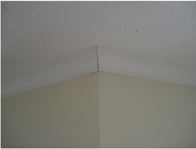
Above: Examples of cracking which would be deemed the maintenance responsibility of the building owner.
