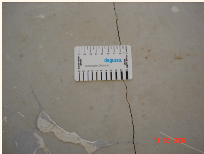
Above: Examples of cracking which would be deemed the maintenance responsibility of the building owner.
