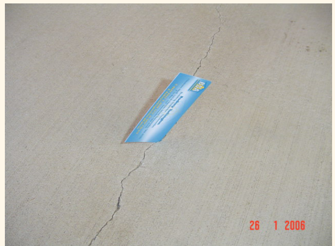
Above: Examples of cracking which would be deemed the maintenance responsibility of the building owner.
